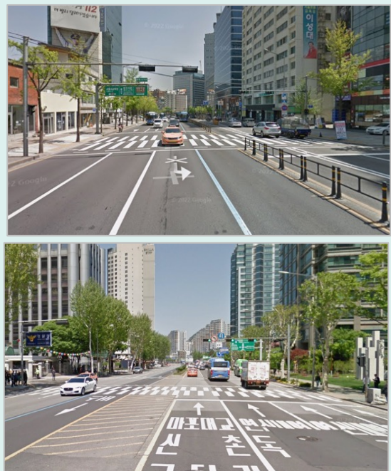
Figure 42: Examples of an at-grade pedestrian crossings on a wide road in Seoul 60
