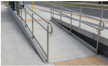
Figure 103: Ramp to accommodate level change 131
