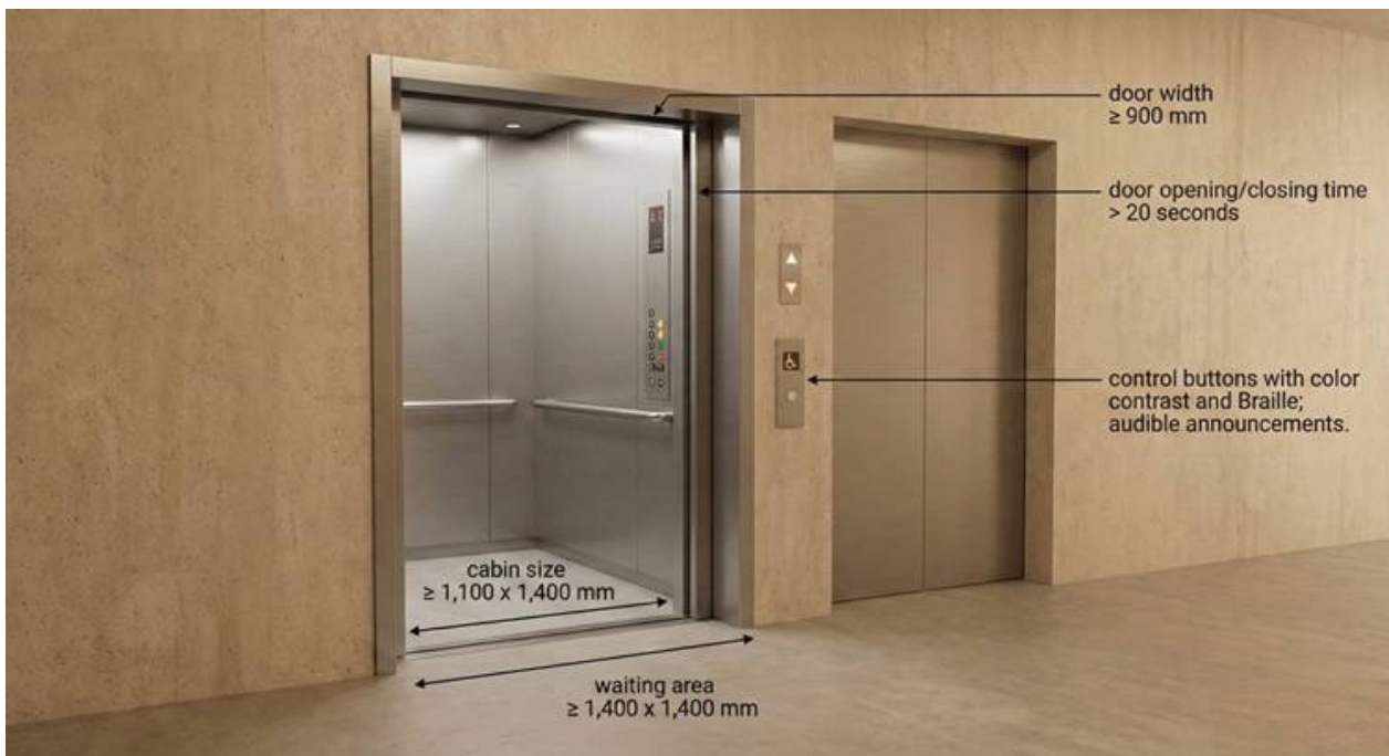
Figure 93: Accessible elevator design 121
