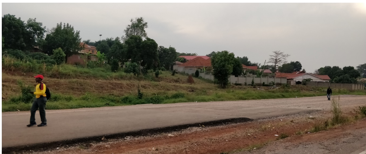
Figure 12 Northern Bypass under construction, Kampala. Photo Credit: Arup
