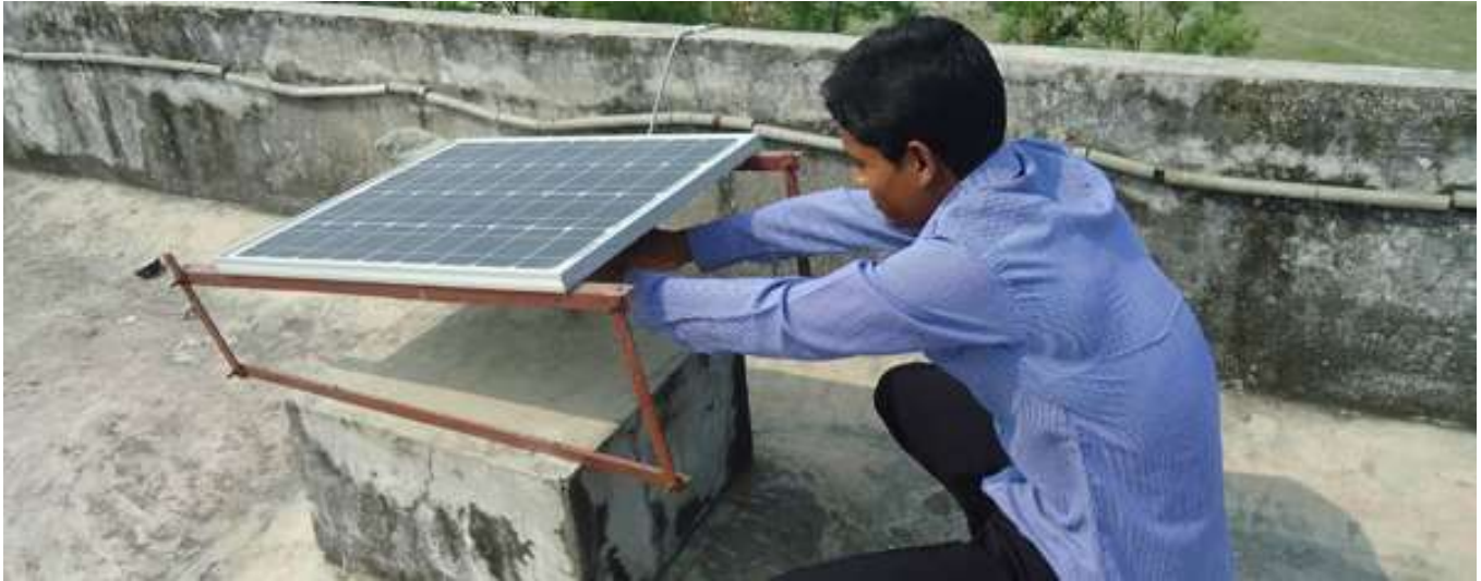
Solar panel installation in Bangladesh. Photo: ILO
